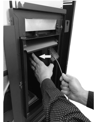
Fig. 71 - Clean with pipe cleaner
